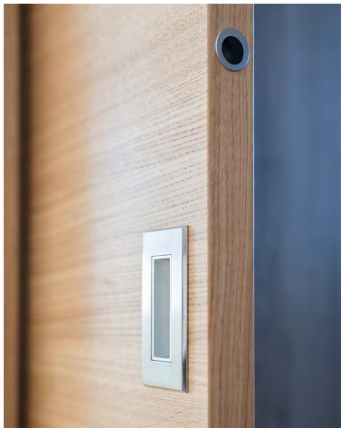
drsna vrata v kaseto s podbojem sliding door in a cassette with a frame
